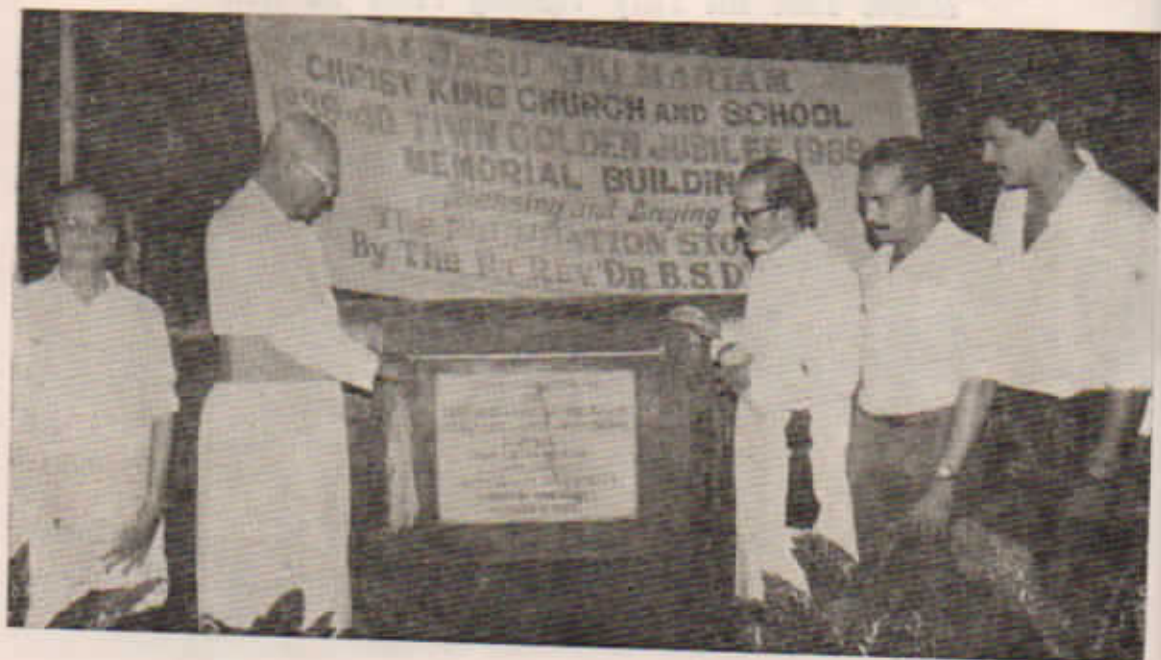
Foundation Laid On Rock
