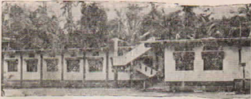
ನನ್ಯಾ ಇಸ್ಕೂಲಾಚೆಂ ಬಾಂದಾಪ್ THE INCOMPLETED NEW SCHOOL BUILDING
